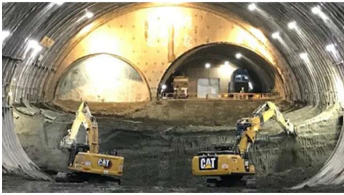
Figure 13. Excavation of the lower half and primary invert
