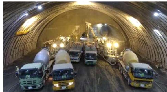
Figure 10. Upper half spraying
