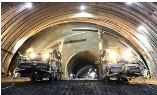
Figure 11. Erection of the upper half steel arch support
