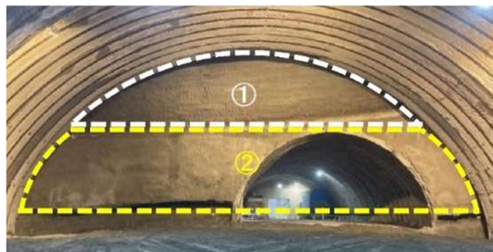
Figure 16. Excavation of the upper half divided in two stages
