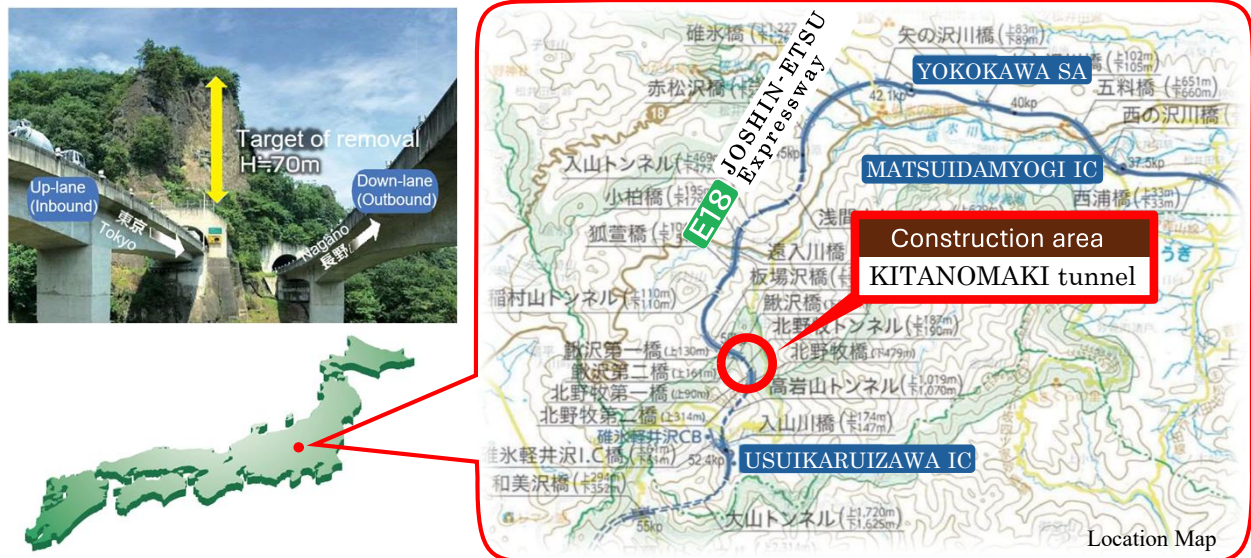
Figure 1. Target slope ( West side of KITANOMAKI-tunnel entrance )
