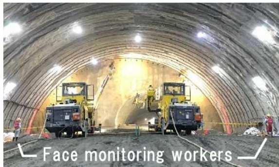
Figure 20. Position of face monitor-ing workers
