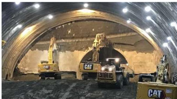
Figure 9. Upper half excavation
