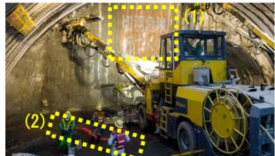
Figure 19. Safety measures in the vicinity of the face
