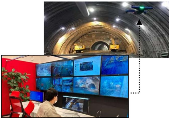
Figure 17. Drone photography and monitoring in safety support room
