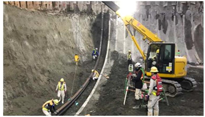
Figure 14. Erection of the lower half and primary invert support
