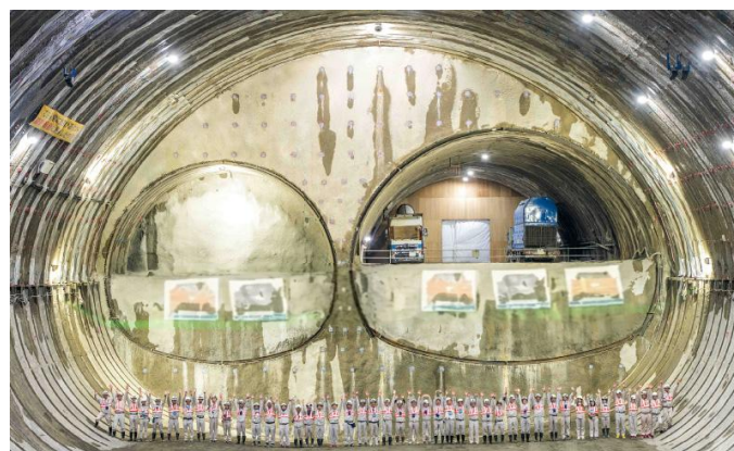
Figure 3. Completed excavation of ultra-large-cross-section
