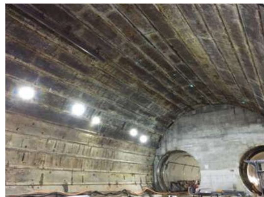
Photo-1 Construction of the tunnel by element propulsion
