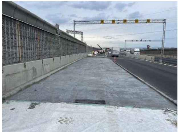
Photo-4 Completion of work
