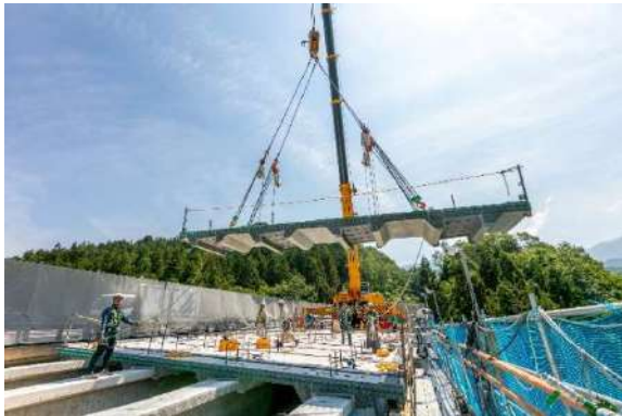
Photo-1 Erection of PCa panels
