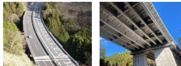
Photo-2 Kamitagawa Bridge
