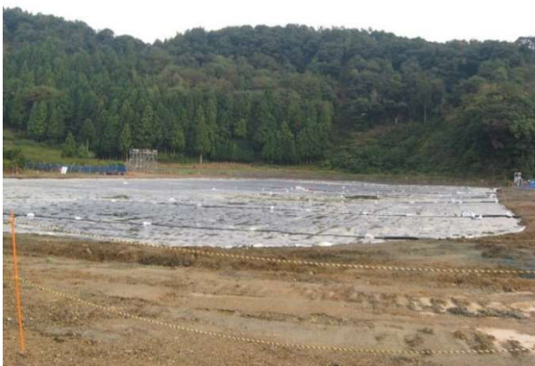
Figure-9 Vacuum Consolidation Area
