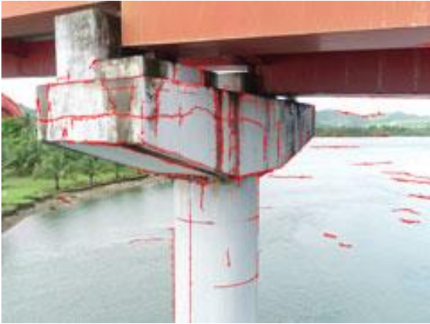
Photo 10. Analysis result of concrete crack
