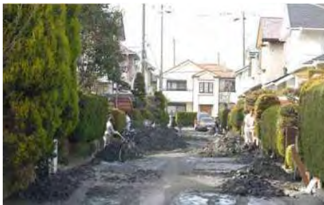
Photo-1: Residential Area Liquefaction caused by the Great East Japan Earthquake
