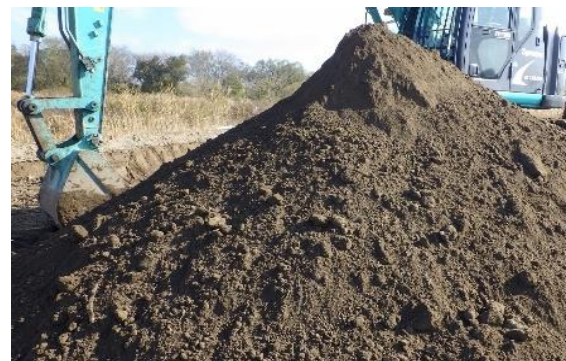
Photo-4 Granulation by loosening
