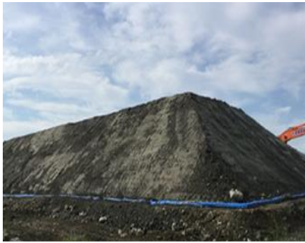
Photo-5 Reusing improved soil for embankment material
