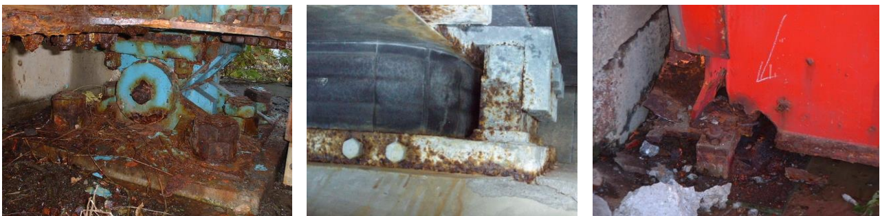
Figure-1 Corrosion of bridge bearings
