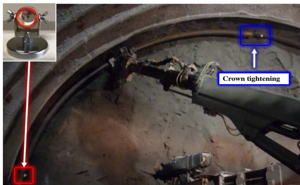
Photo-3 Crown tightening, and positioning of the steel timbering
