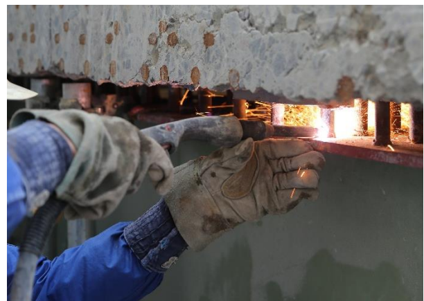
Photo-3 Cutting the stud
