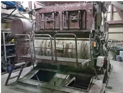
(b) Concrete batching plant
