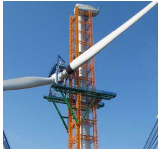
Figure 6 Rotor Assembling
