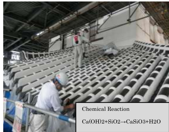
Photo7 Spraying Water Absorption Inhibitor
