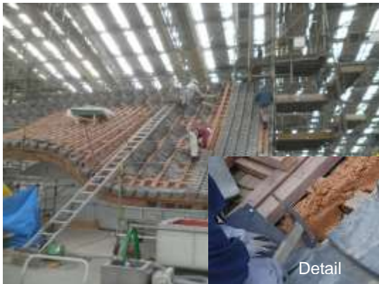
Photo5 Combination Method of Roofing Soil and Wood
