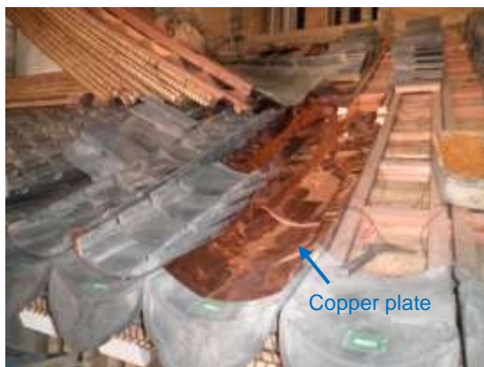
Photo6 Copper plates under roof tiles
