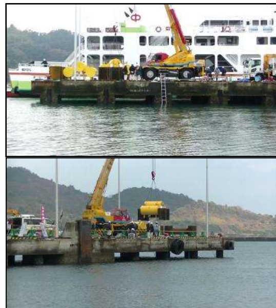
Photo-2. Retrofitting while using a piled pier
