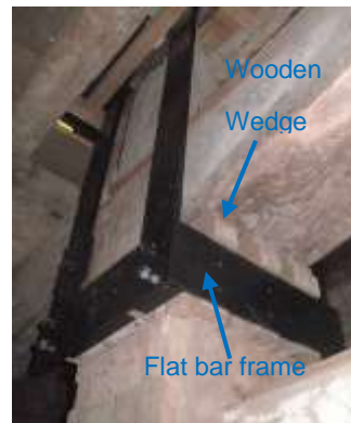
Photo8 Seismic Retrofitting for wood parts
