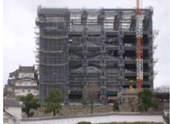
Photo2 Dismantling Process of the Protective Roof Scaffolding
