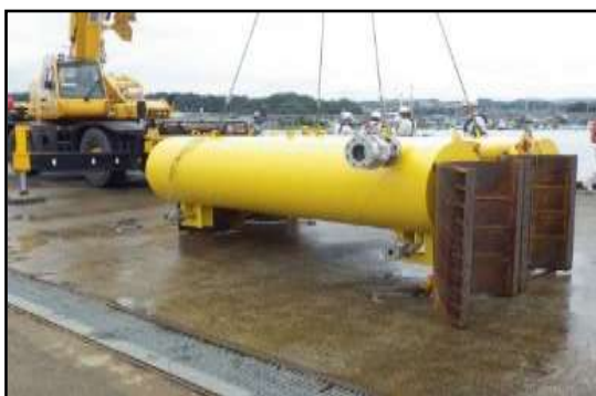
Photo-3. Float specifically designed for the stiffening members
