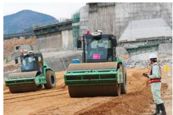
Fig. 3 Automated vibration rollers.
