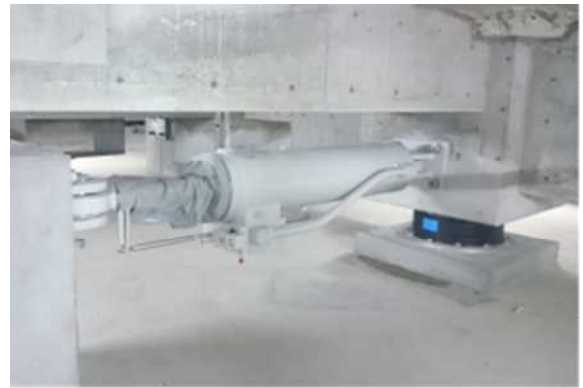
(b) Passive-Switching Oil Damper
