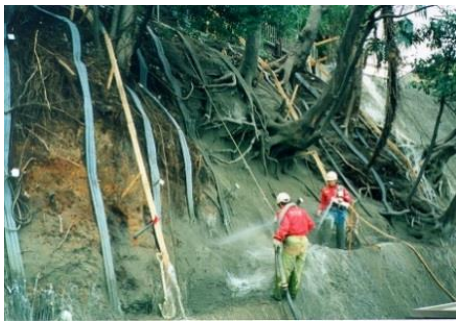
Photo 3 Building a layer of continuous fiber reinforced soil
