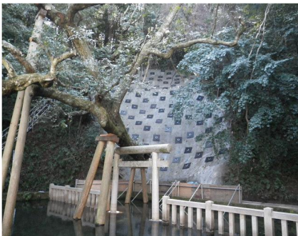
Photo 8 Completion of soil nailing and the continuous fiber reinforced soil layer
