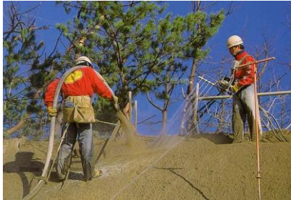
Photo 1 Building a layer of continuous fiber soil (Manual type: sandy soil at left and continuous fiber at right)
