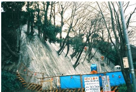
Photo 4 Completed layer of continuous fiber reinforced soil
