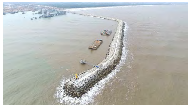
Photo3. Breakwater at NSRP Complex
