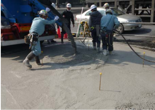
Photo 4 Pavement using sea water and steel slag
