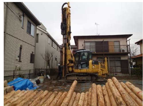
Photo1 Installation by small construction machinery at a narrow site
