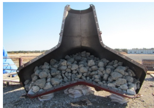
Photo 3 Wave dissipating concrete block using sea water and debris
