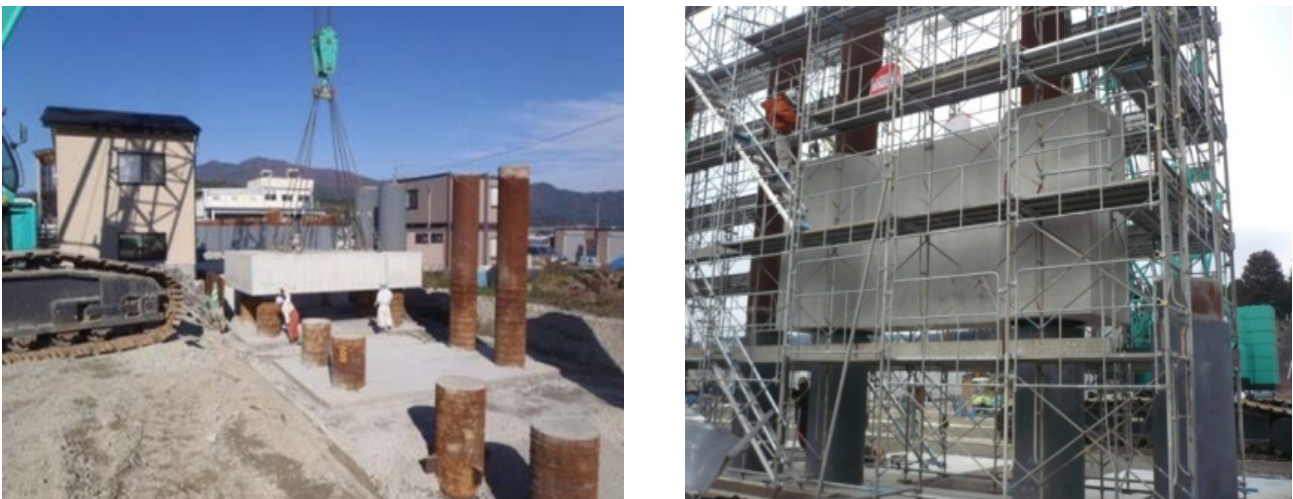
Fig.5 Insert a footing block (left) and a wall block (right) to pre-driven piles for the 1 st disaster restoration construction at Yamada fishery port
