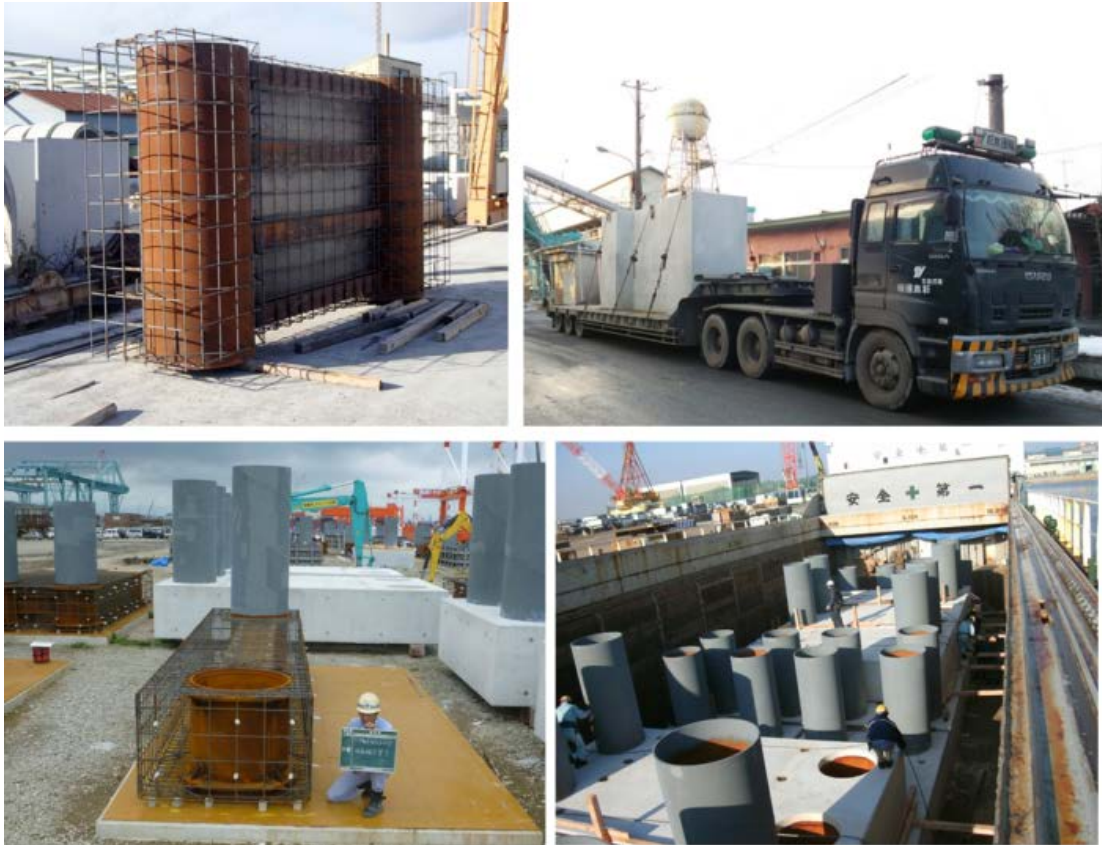
Fig.4 Layout of reinforcement and transport of wall blocks (upper) and footing blocks (lower) for the 1 st disaster restoration construction at Yamada fishery port
