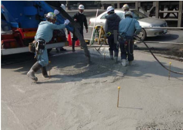
Photo 4 Pavement using sea water and steel slag
